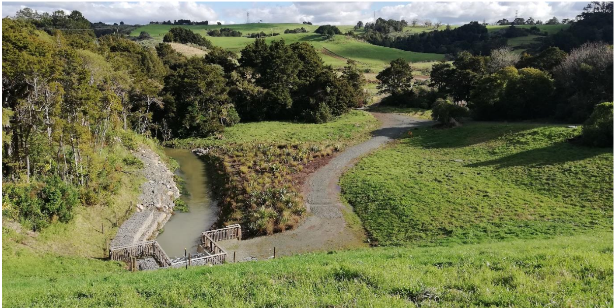
Appendix 14: Hopua te Nihotetea retention dam in normal condition and during the July 2020 event.
