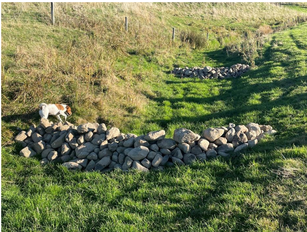
Figure 17. An example of interception of runoff along an ephemeral pathway (swale) in a paddock. Here, a daisy chain (there are three of these structures in a row, one is hidden from view) of boulder check dams was placed within an ephemeral pathway. Jack Russel for scale (courtesy of Chris and Andrea Bullied, Waimea Catchment Group).
