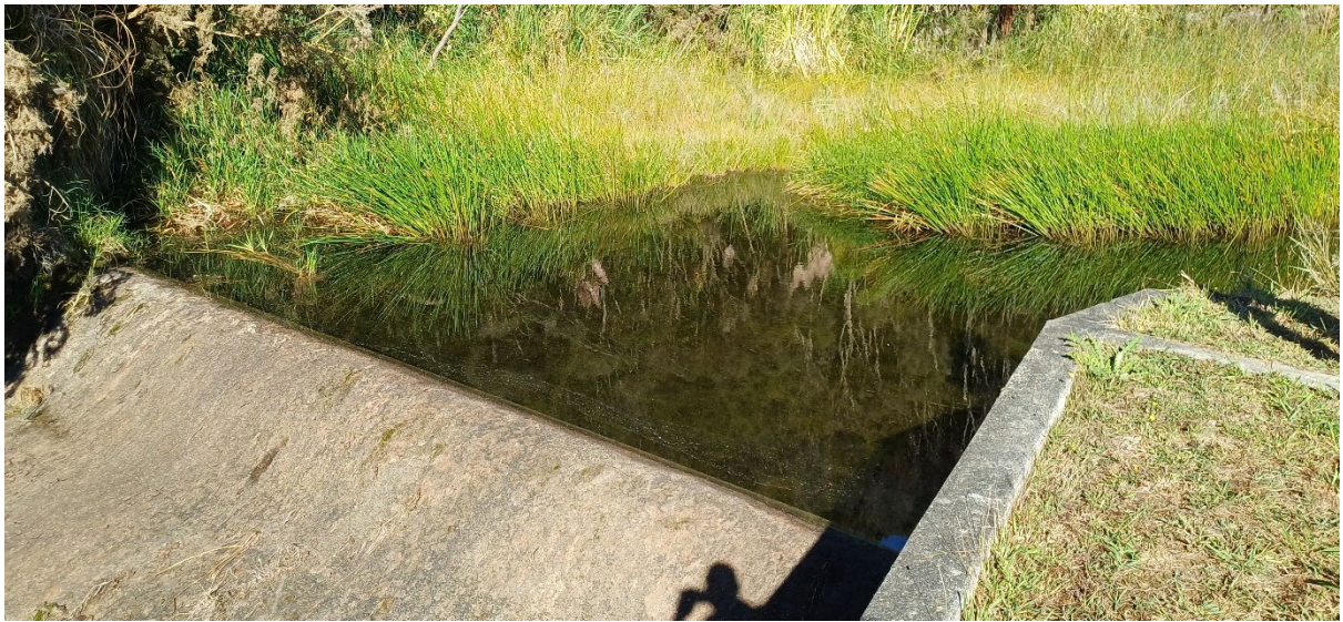
Takahiwai Dam at Outfall (Whangārei Harbour catchment)
